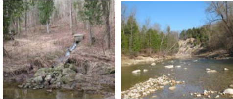
Outfall discharge at side channel
